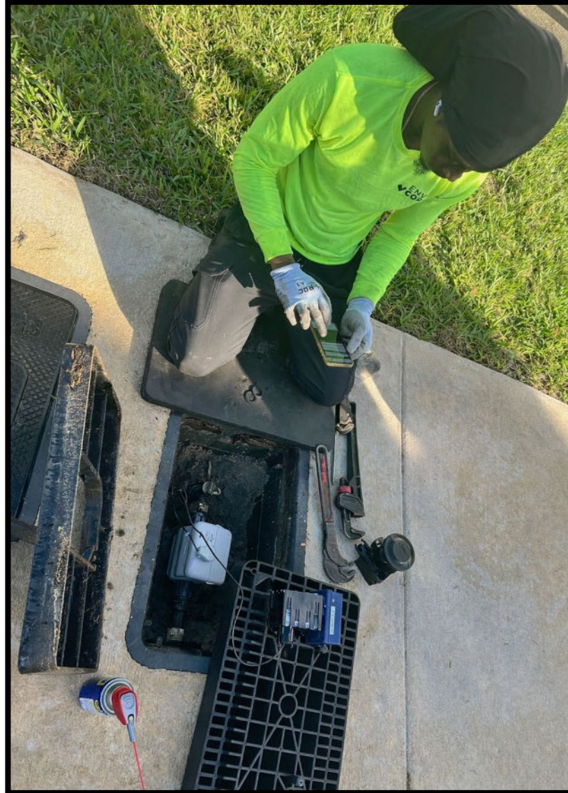
Installation and activation
