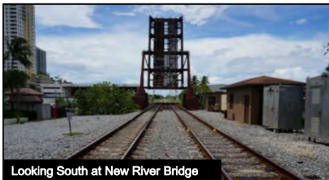
Looking South at New River Bridge
